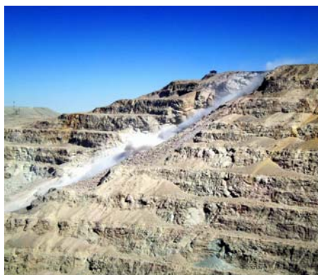
Gentek's work at Mountain Taurus West Copper Mine includes stabilizing a large landslide by designing an economical flexible pin system (shown at left) that anchored the upper sliding mass to the lower sliding mass. (Picture before operation)
