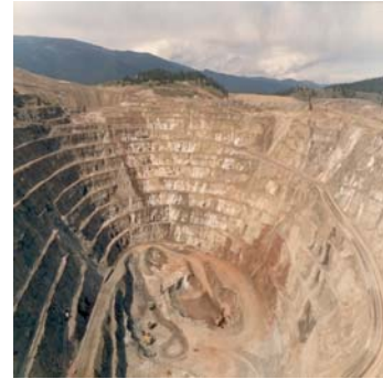
Gentek performed slope stability and transient seepage analyses for Dewatering this large open-pit iron mine in soil and rock. (Soganli Mountains, Turkey; Client : Blacksea iron company)
